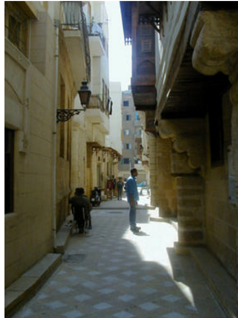
Fig. 4, Good quality of preservation in Al-Darb Al-Asfar for buildings, but with no economic activities.
